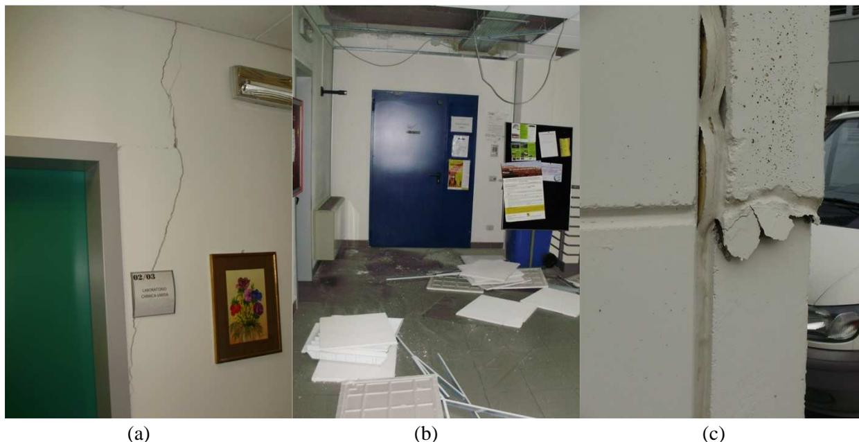
Figure 3 – Damage occurred on the SDT side of the investigated building. (a) curtain wall of the chemistry laboratory at the ground floor; (b) SDT side entrance at the second floor; (c) detail of one of the external wall.
